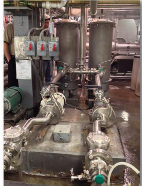
Stage 1: Backwash frequency is based upon PSID or time at the direction of the Plant Manager. SOP is to replace cartridges every 6-12 months.
