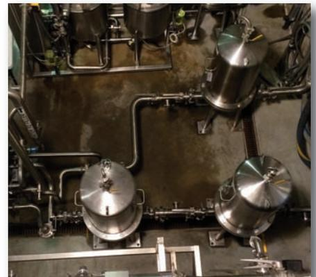
Existing PES .6 um stage 1 (lower right vessel) and .2 um stage 2 PES filters (lower left vessel) were replaced with .45 um absolute backwashable filters in stage 1 and Charged Membrane Filters in stage 2. The 2.5 x 30 inch cartridges were designed to fit exiting filter vessel making the change out steamless to product line.
